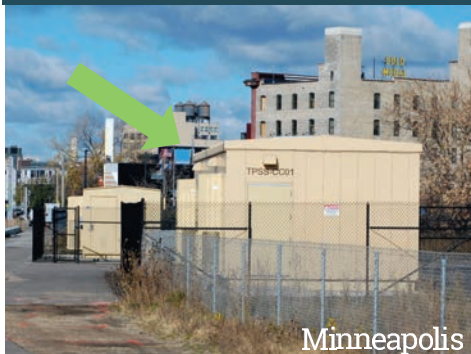
Traction Power Substation
